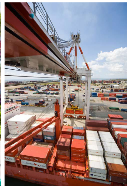
Port of Brisbane A Cbus infrastructure investment managed by IFM.
