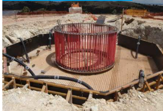
ROCK ANCHORED FOUNDATION
