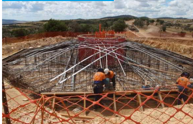
ROCK ANCHORED FOUNDATION
