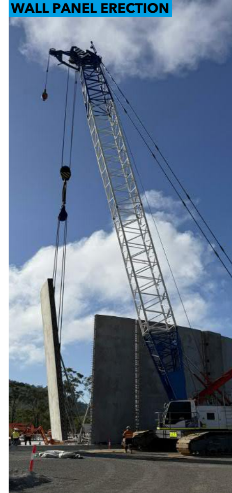
WALL PANEL ERECTION
